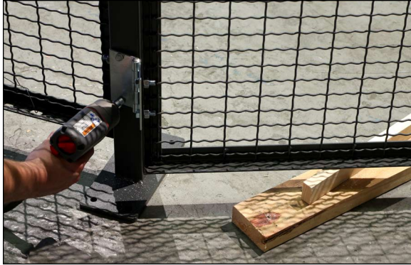
Attach bottom door hinge to post with self-tapping screws.
